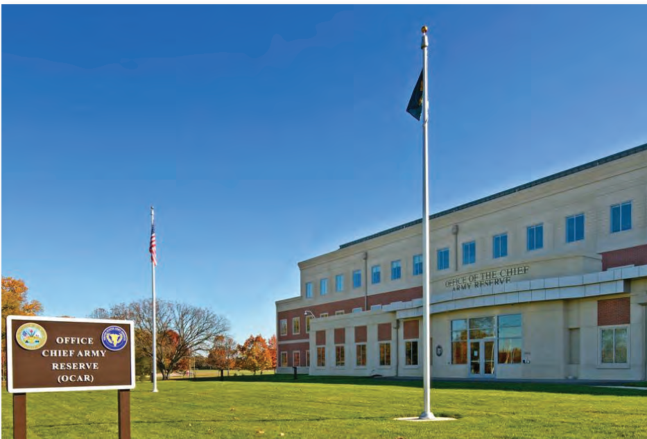
Office of the Chief Army Reserve headquarters at Fort Belvoir, Virginia.
